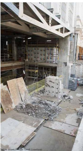
The transformation of the main foyer at ground level is at the heart of the changes being made, and earlier this year, work began to remove the concrete piers holding up the cast-iron and glass structure that is the impressive Paul Hamlyn Hall. This means that from 2018 the public will be able to see into the building from Bow Street across an expansive foyer and down into the Linbury Theatre.
