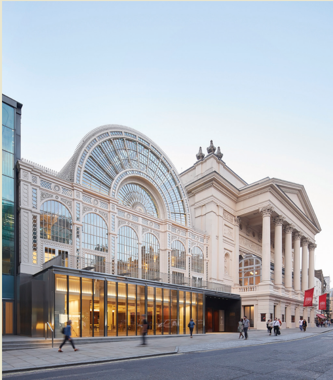
Bow Street Entrance
